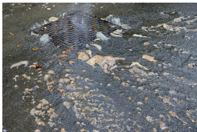
Foul sewer discharging in The Lane Chilton 4 th Feb 2014 due to overload of waste water drainage system (NOT blockage).
